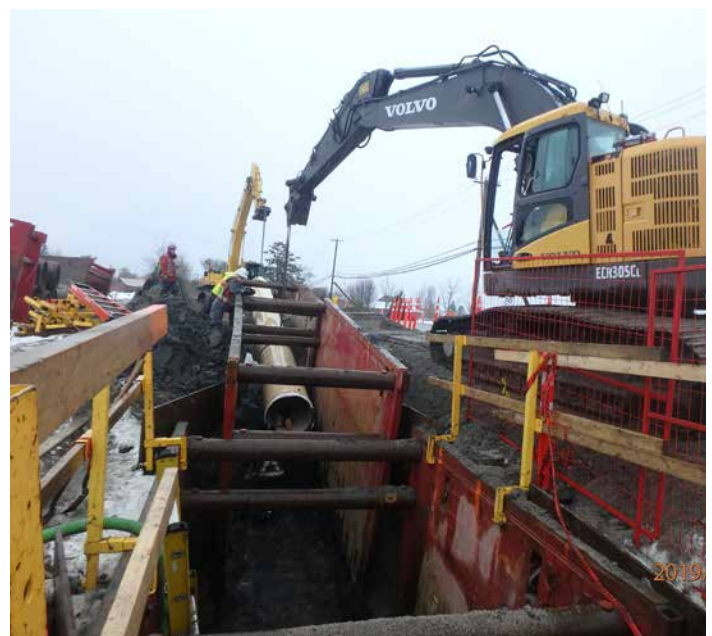
Crews installing a new water main pipe into a trench
