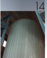
Lime and carbon are added to the cooled flue gas (i.e. gas exiting to the atmosphere via a flue or stack as it's known at the Facility) to react with acid gases and vaporous metals allowing them to be captured.
