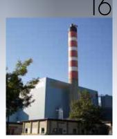
The filtered air exits the Facility though a stack with continuous air emissions monitoring. Independent stack testing is also done.
