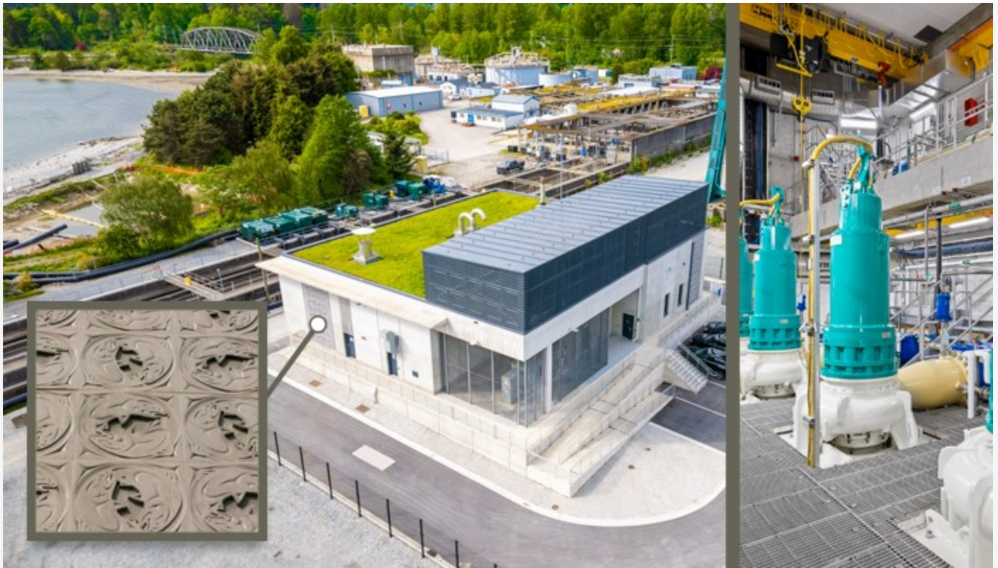
The newly constructed First Narrows Pump Station, located under the Lions Gate Bridge (exterior – left image; interior pumps and equipment – right image) will help to move wastewater from West Vancouver to the new North Shore Wastewater Treatment Plant. The building façade features original artwork by James Harry (commissioned by North Shore Conveyance Partners and Metro Vancouver – see inset). Kenaidan Contracting Ltd., received a Vancouver Regional Construction Association 2022 Award of Excellence for their work on the pump station.
