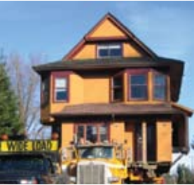
Photo courtesy Nickel Bros. House Moving Ltd.
