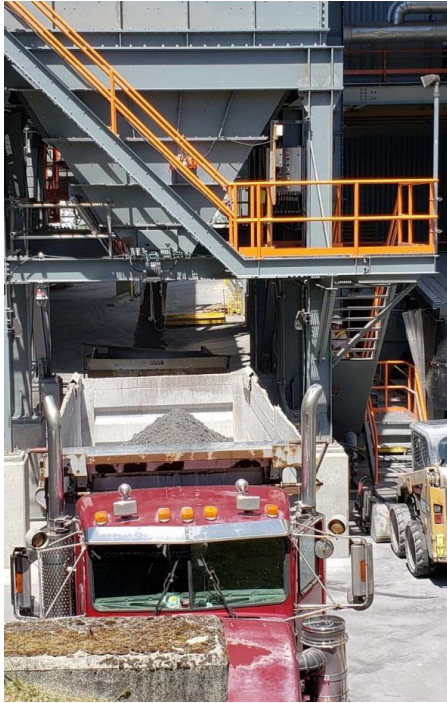
Bottom Ash Loading
