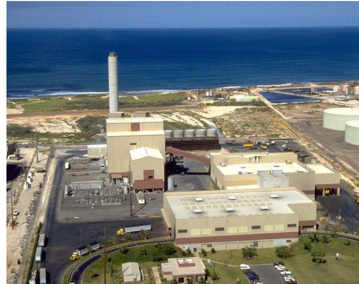
H-POWER Waste-to-Energy Facility, Honolulu, Hawaii
