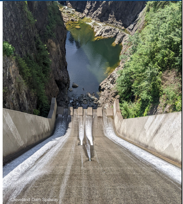
Cleveland Dam Spillway
