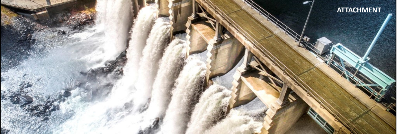
Seymour Falls Dam Spillway
