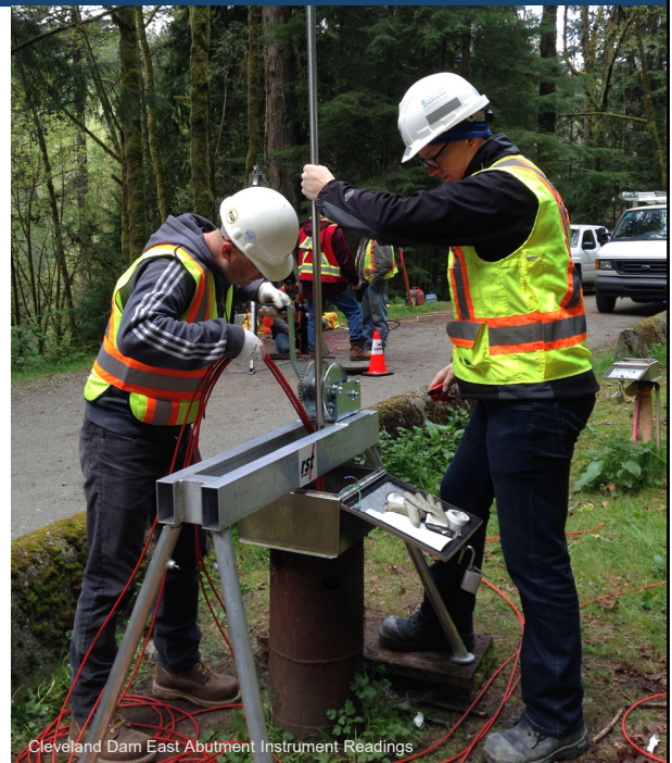
Cleveland Dam East Abutment Instrument Readings
