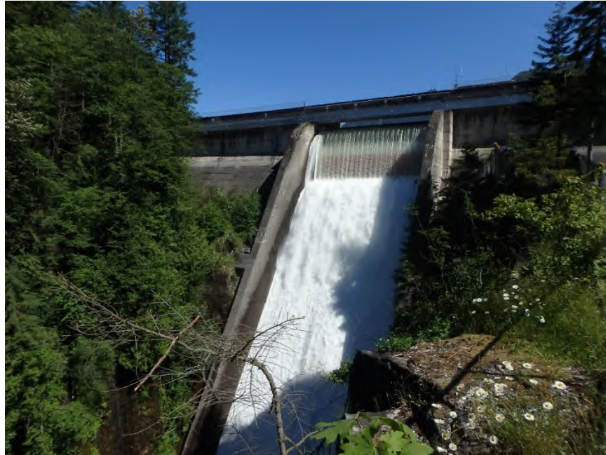
GVWD Water Supply Dams: Cleveland Dam
