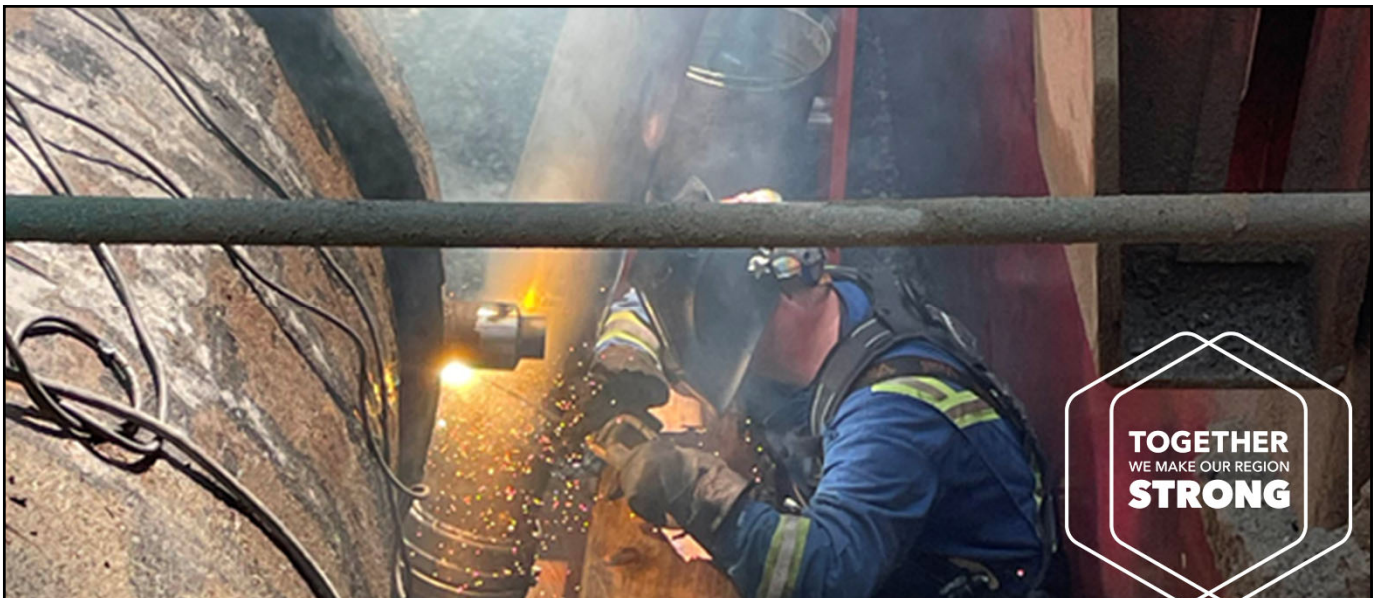
Capilano Main No.4 2023 Leak Repair – Welding of Permanent Repair
