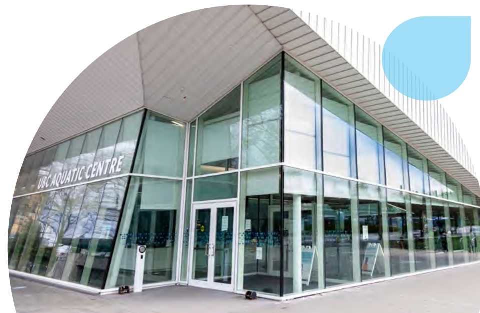
The UBC Aquatic Centre demonstrates a multi-use facility that supplies non-potable water that meets toilet flushing and recreational water standards.
