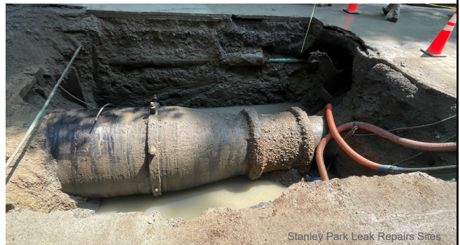
Stanley Park Leak Repairs Sites
