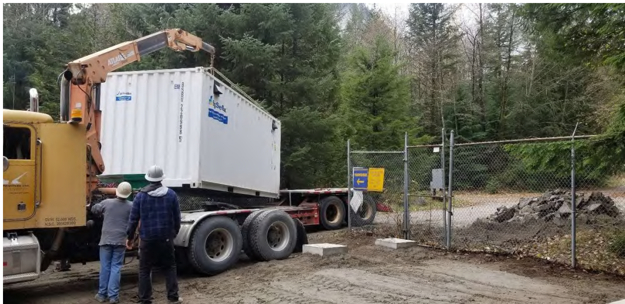
FIGURE 14 INSTALLATION OF FITTED-OUT FEED STORAGE CONTAINER
