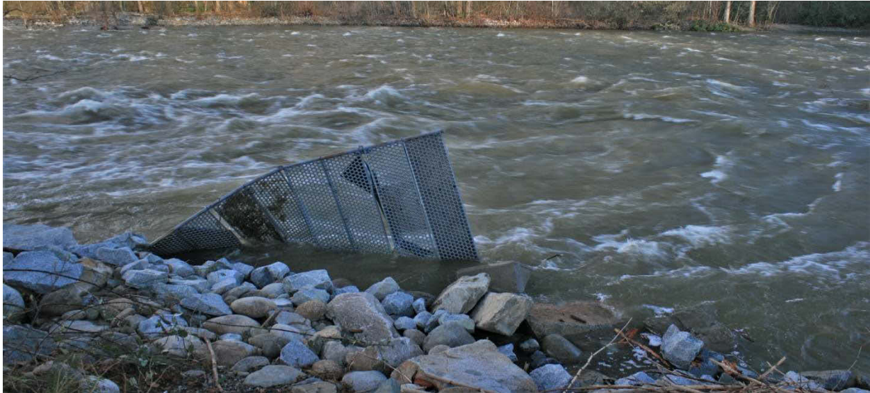
FIGURE 14 DAMAGED FISH FENCE FOLLOWING HIGH FLOW EVENT
