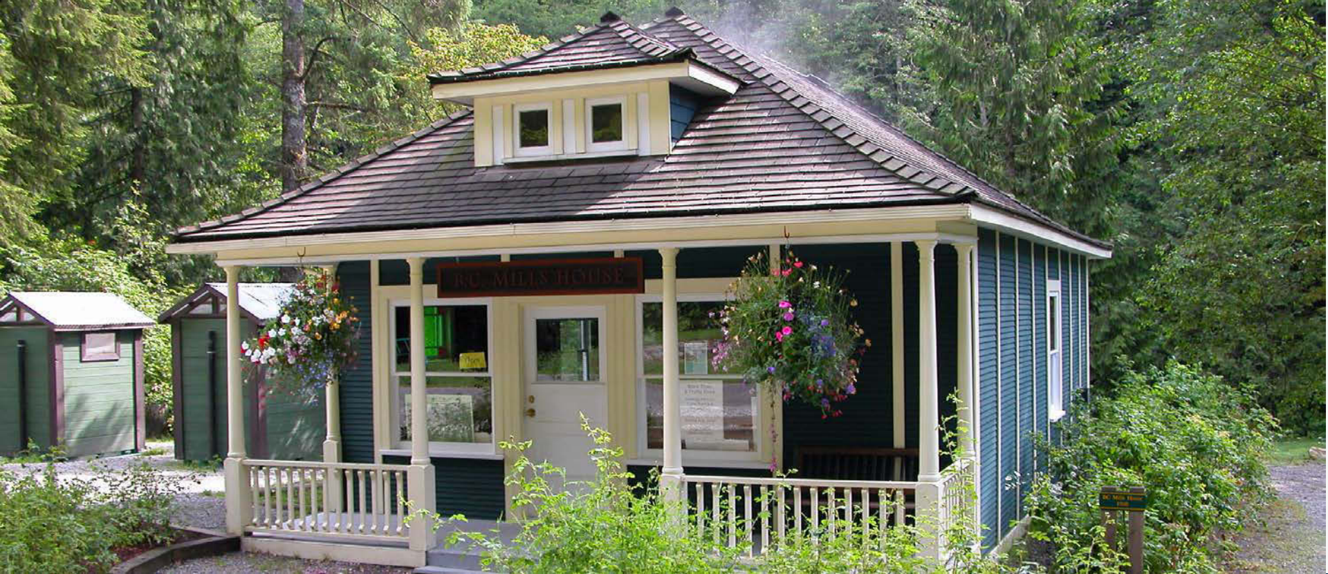
B.C. Mills House & Pit Toilets, Lynn Headwaters Regional Park
