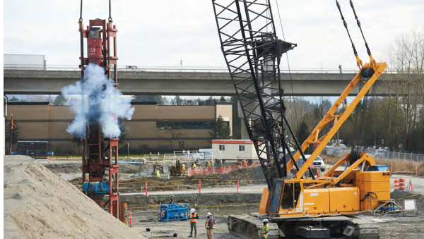
Early works ground improvements
