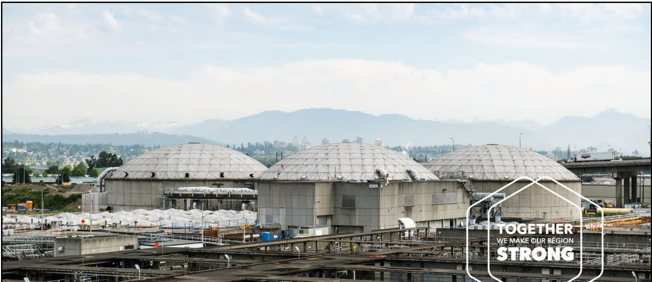
Annacis Island Wastewater Treatment Plant Tricking Filters
