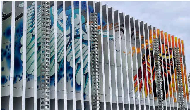
Pump Station & SSO Tank – Katzie artist Rain Pierre
