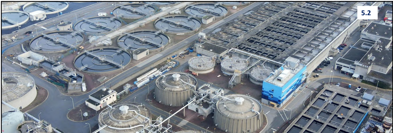
Annacis Island Wastewater Treatment Plant
