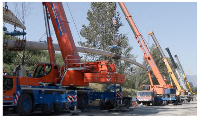
Fraser River Crossing – Installation of first pipe
