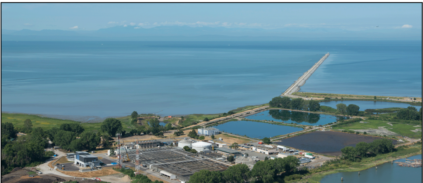
Iona Island Wastewater Treatment Plant
