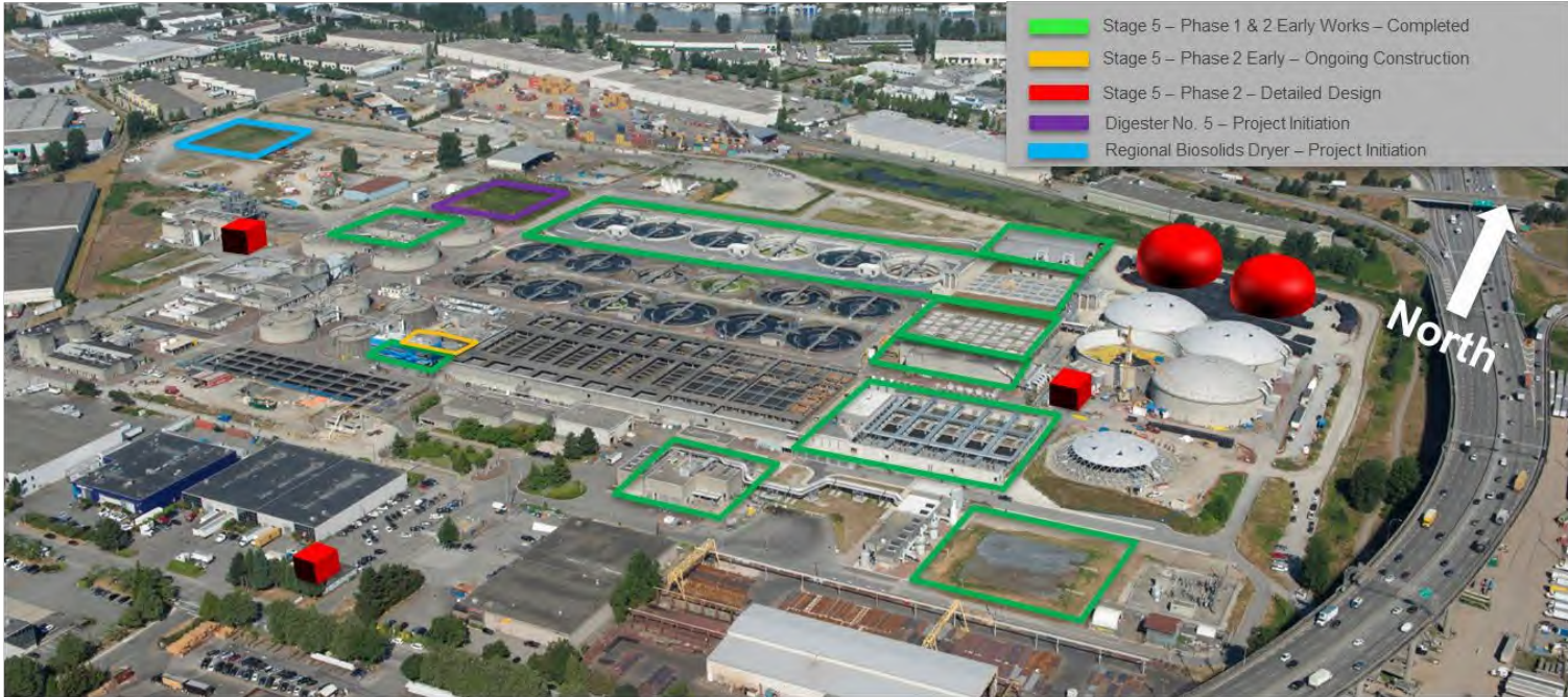
Annacis Island Wastewater Treatment Plant
