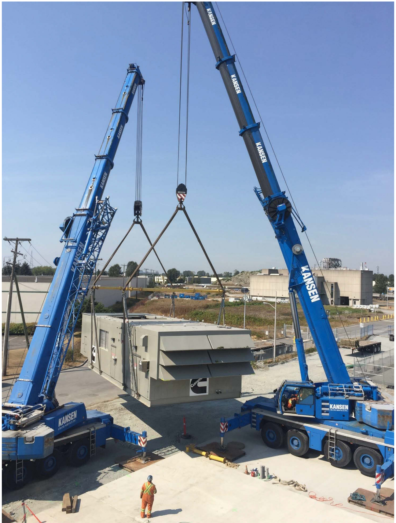
Delivery of One of the Two 3 MW Diesel Backup Power Generators
