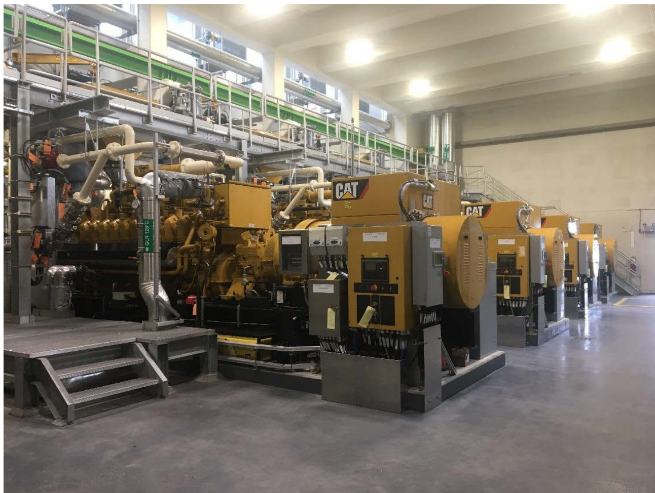
Four New 2 MW Cogeneration Engines
