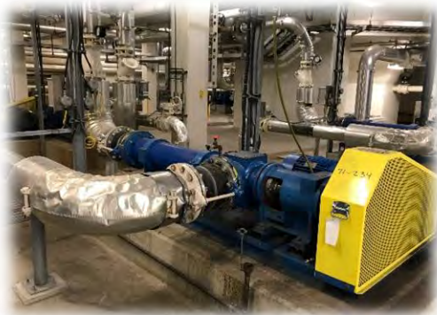
Additional Mixed Sludge Feed Pumps to improve redundancy and meet future capacity
