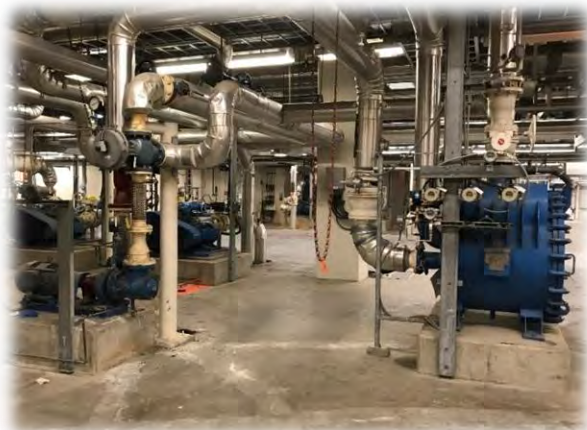
Additional Circulating Sludge/ Heating Reservoir Supply Heat Exchangers with associated Hot Water Circulation Pumps and Digested Sludge Circulation Pumps to meet future capacity
