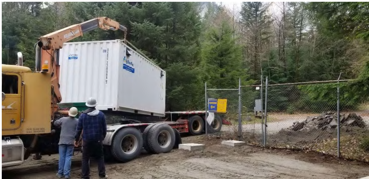
FIGURE 14 INSTALLATION OF FITTED-OUT FEED STORAGE CONTAINER
