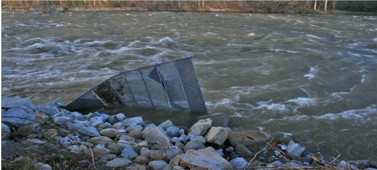
FIGURE 14 DAMAGED FISH FENCE FOLLOWING HIGH FLOW EVENT
