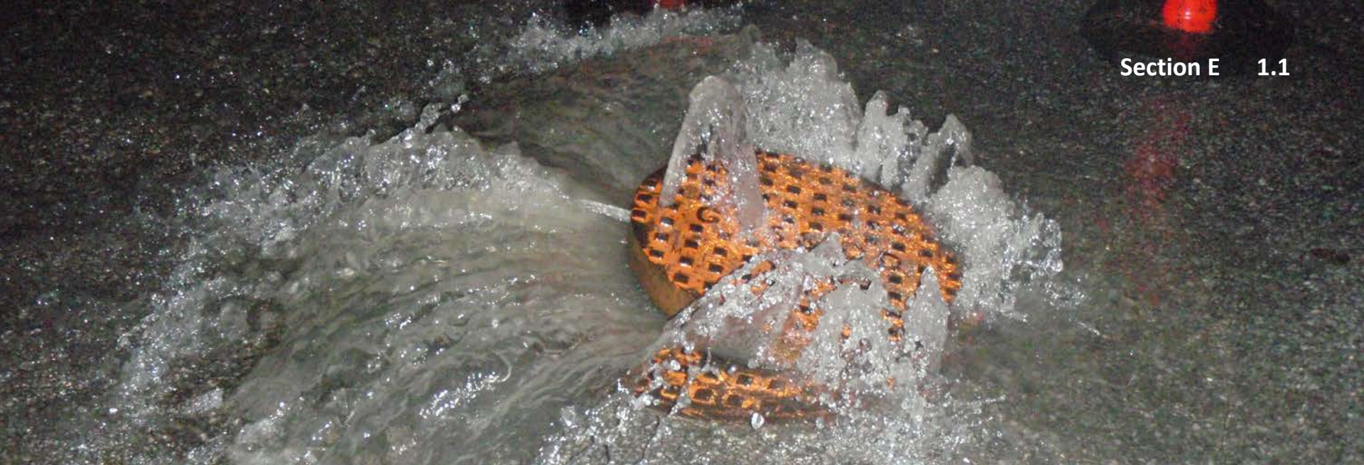
Sanitary Sewer Overflow
