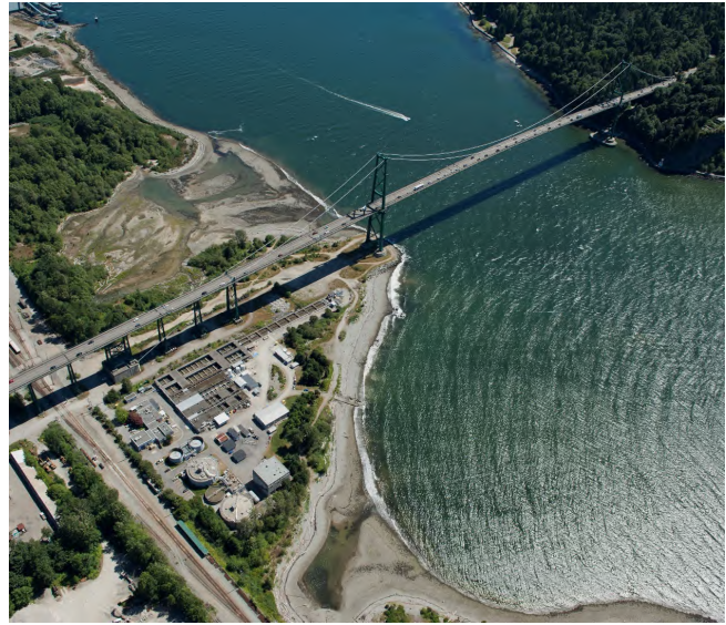
Lions Gate WWTP and Lions Gate Bridge, 2013
