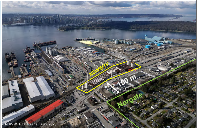
NSWWTP Site aerial, April 2023
