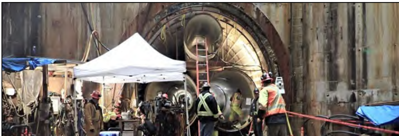
Second Narrows Water Supply Tunnel
