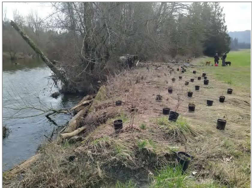
Figure 1. Planting native species to stabilize riverbank on agricultural land. 1
