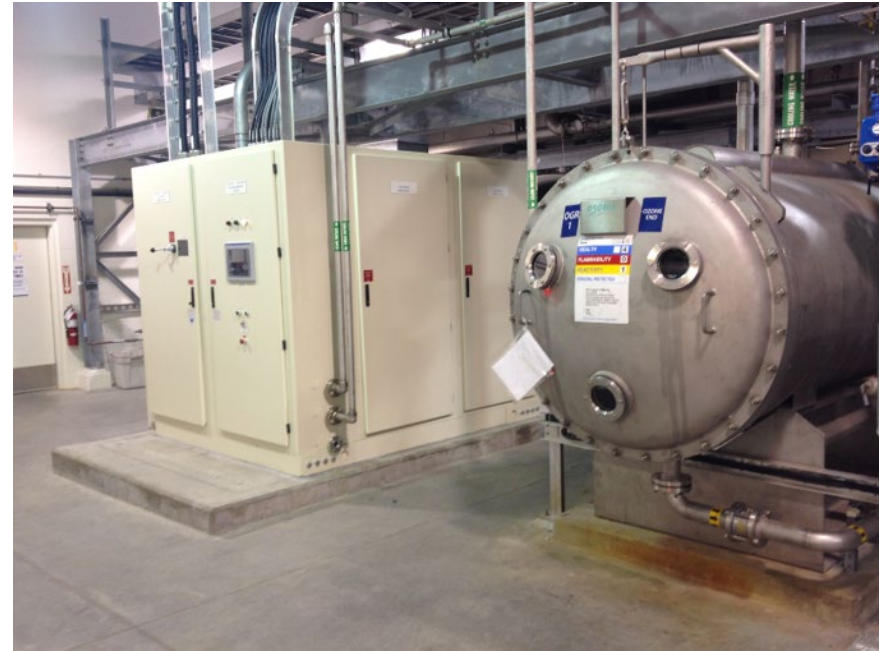
Ozone Generator at the Coquitlam Water Treatment Plant
