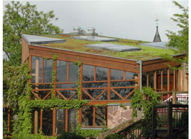
Extensive green roof – Halle Zoo, Germany
