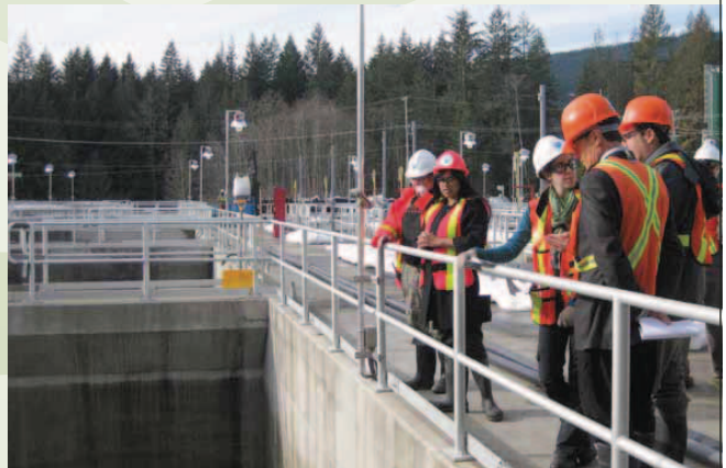
Tour of the SCFP – Flocculation area
